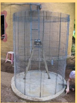
Ferrocement Tank
